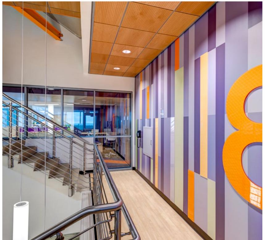
Together, the fire-rated glass and frames offer fire ratings of up to two hours and block the transfer of radiant heat. They provide essential protection should faculty or patients need to exit the building during a fire.
